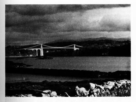
Menai Bridge from the Anglesey shore This photograph shows the steel chains which replaced the original wrought iron in 1938. The wall of an old fish trap can be seen in the foreground. (Photograph: Elisabeth Beazley)
