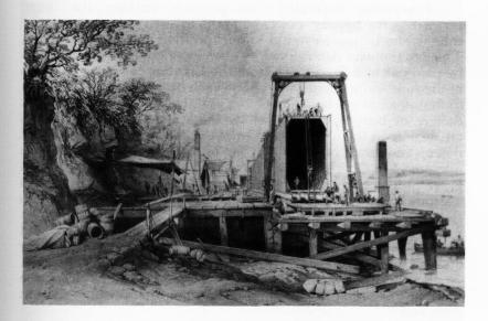
Britannia Bridge. Platform & construction of the tubes, September 1848. (Engraving by G. Hawkins)
